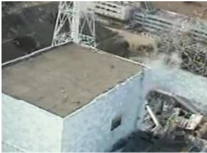
Steam Coming Out From Blow-out Panel (4/10/2011)
