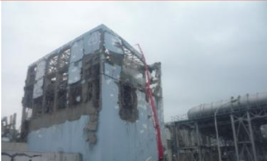
Water Injection by Concrete Pumper (3/22/2011)
