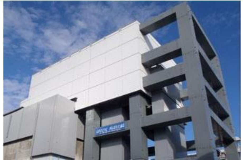
Fuel Removal Structure (Nov. 2013)
