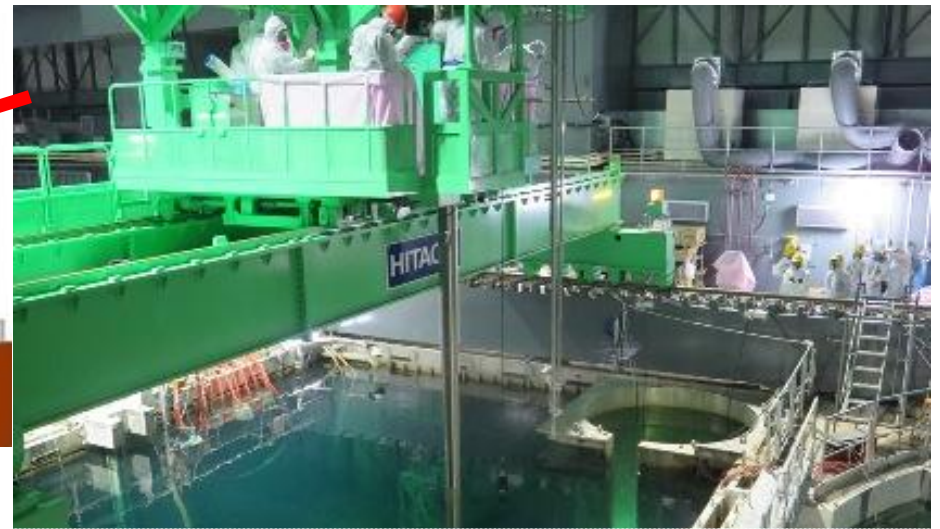
Fuel Removal from SFP (11/18/2013)
